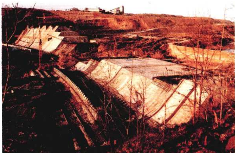
3. Dam Construction site, Indira Sagar Project, M.P.
