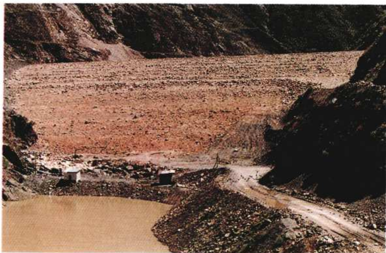
a) Raising of Cofferdam upto 661m
