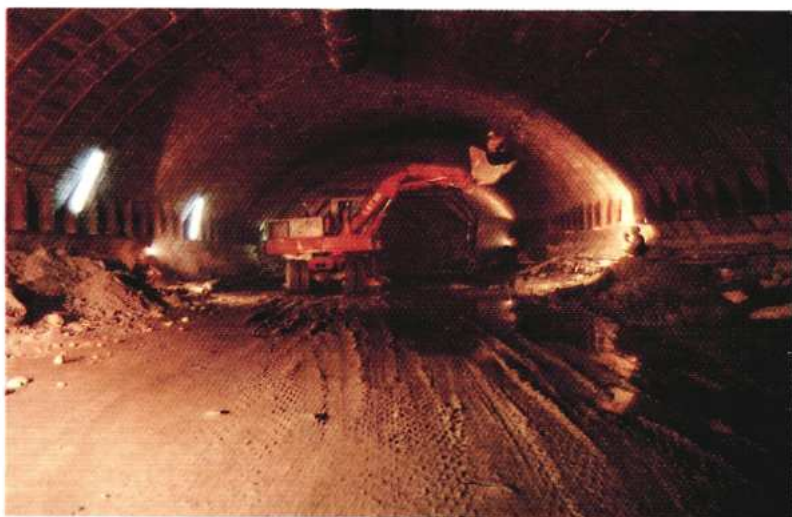
b) Power House Construction Work at Tehri Dam Project Site
