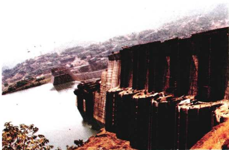
4. Intake portion for Right Bank Power House of Sardar Sarovar Project, Gujarat
