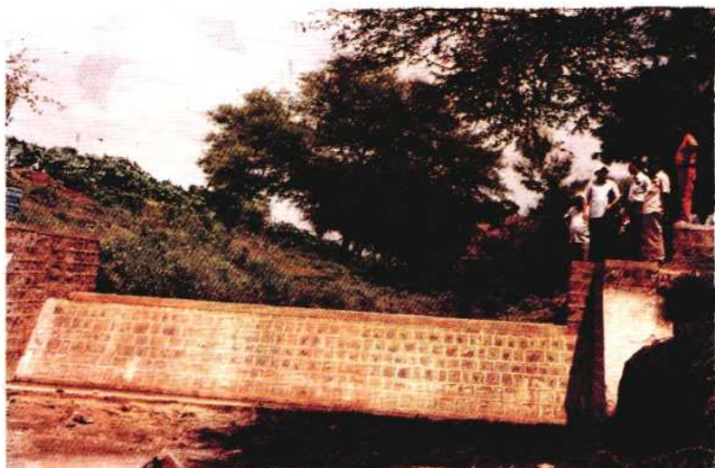
6. Stream Runoff Management Structure in District Manawar, M.P.
