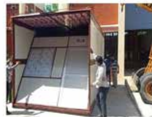
Opening of front and back door panels
