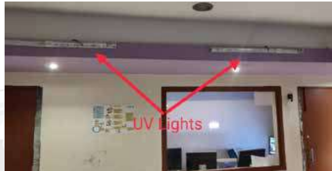
CT room with installed UV lights
