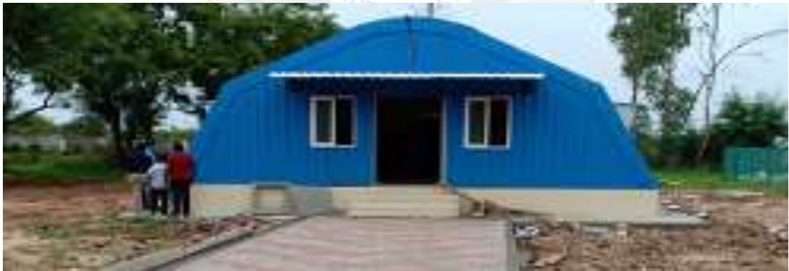
Stages of Construction: 10-Bed Makeshift Hospital at NDRF, Arakkonam
