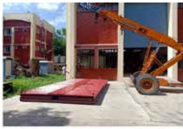
Initial position (transported to site in complete foldable form)
